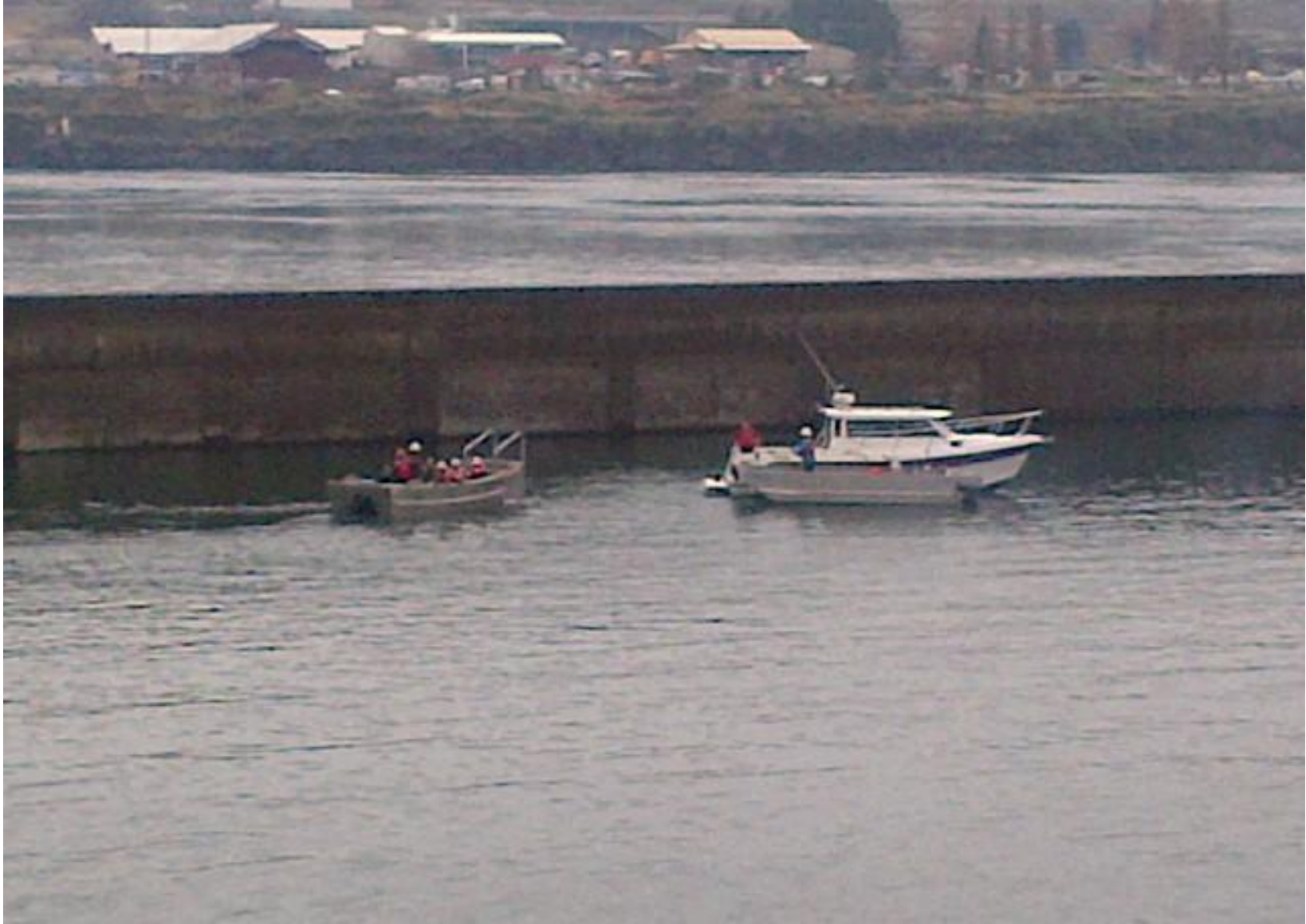
Contractor divers completing minor repairs to spillwall.
